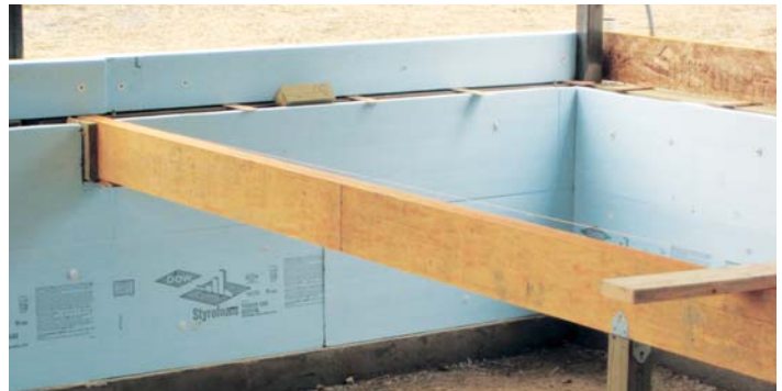
Figure 5. The new footings (above) and stem walls (above right) were formed and poured around the steel columns. The foundation and rim joist were carefully insulated with 2-inch polystyrene (right).
