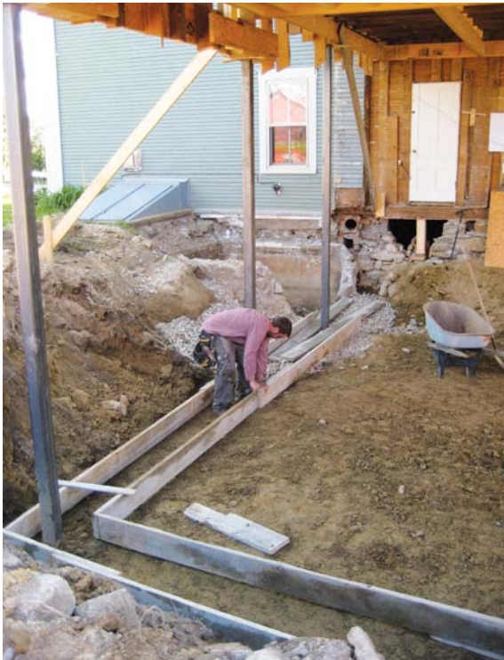
Figure 5. The new footings (above) and stem walls (above right) were formed and poured around the steel columns. The foundation and rim joist were carefully insulated with 2-inch polystyrene (right).
