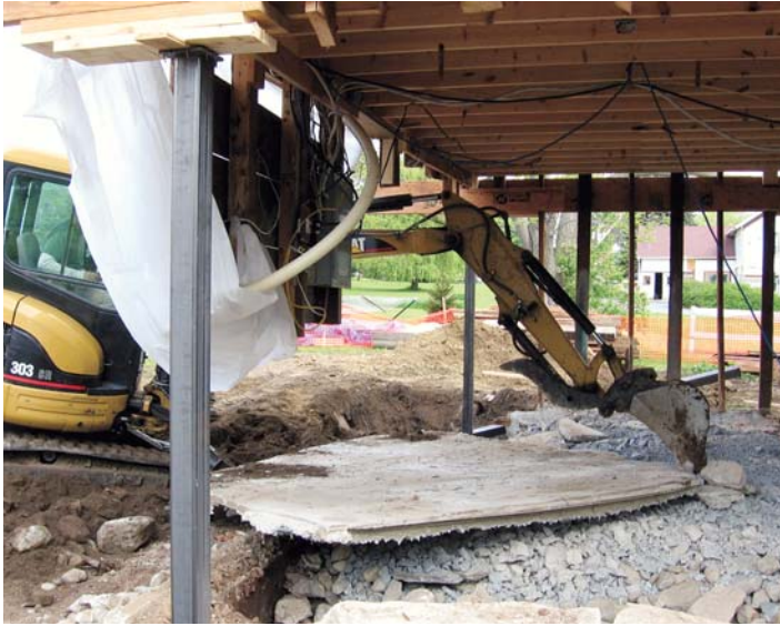
Figure 4. With the walls out of the way, the excavator carefully removes an existing concrete slab (above); part of the foundation had to be jackhammered into submission (right).
