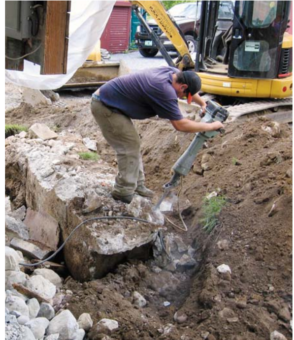
Figure 4. With the walls out of the way, the excavator carefully removes an existing concrete slab (above); part of the foundation had to be jackhammered into submission (right).
